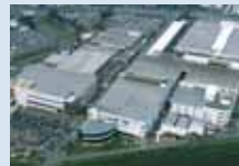
Malacca, Malaysia ○ Power semiconductors, discrete semiconductors, sensors, ICs, package development
