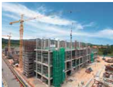
Second manufacturing building in Kulim (Malaysia) shortly before the topping-out ceremony
