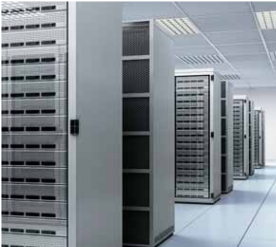
POWER MANAGEMENT & MULTIMARKET
